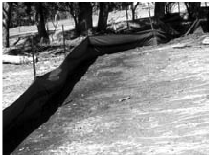
Where containment areas are close to dams, or water ways, silt traps are required to protect dam or stream water quality
